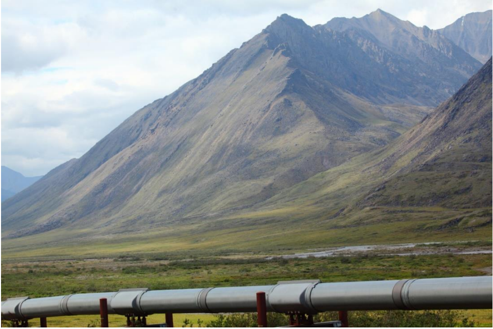
Pipeline at Tea Lake with Brooks Range in background
