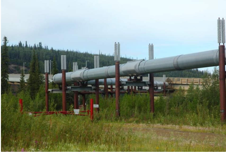
The pipeline just after crossing the Yukon River
