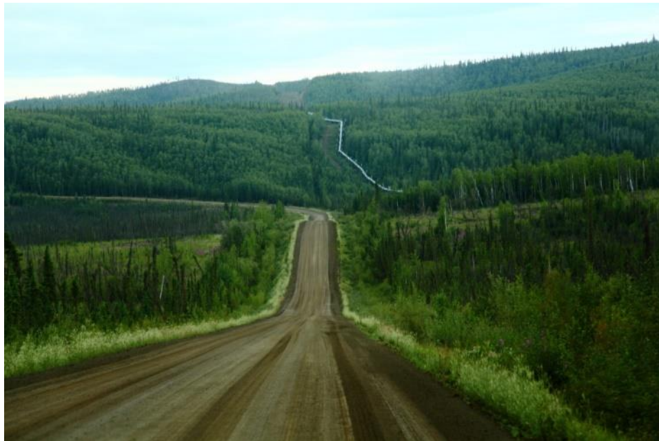
Gravel section of Dalton Highway with view of oil pipeline
