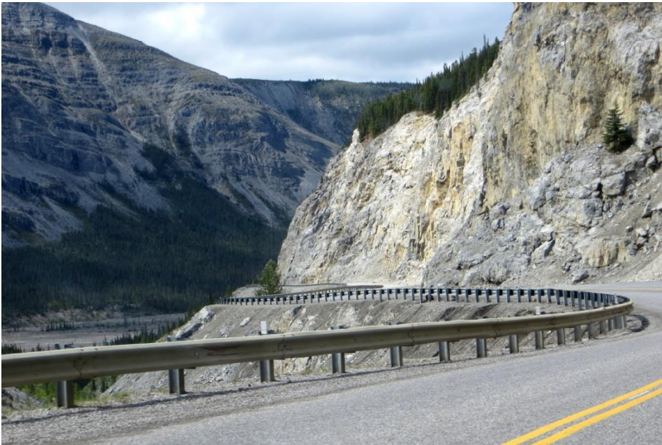
Alaska Highway through Stone Mountain Provincial Park
