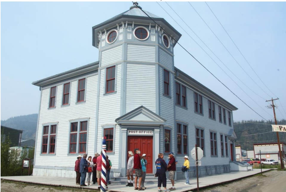
Restored Post Office
