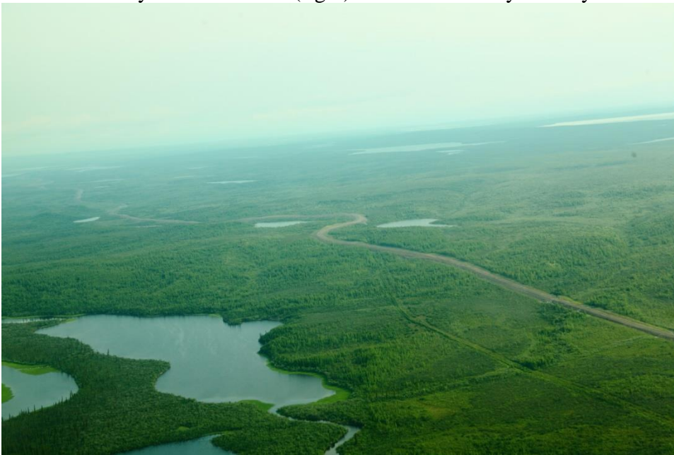
New highway under construction to Tuk, here through taiga
